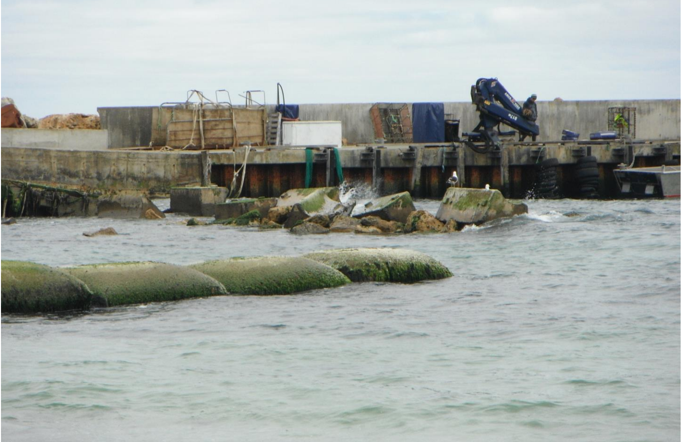
Below: Landward end of Pitt Island wharf, and the breakwaters.
